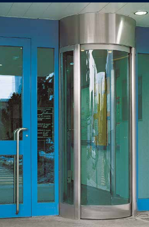
Circular booth as a night time entrance to an administrative building beside the main entrance.
